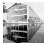
Private Building (Project) Industrial Building. Tsingtao Beer. (Qingdao, Shandong, China)
