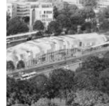
Public Building (Project) Metro Station. Line 6. (Qingdao, Shandong, China)
