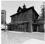
Public Heritage Building (Under construction) Metro Station. Line 4. (Qingdao, Shandong, China)
