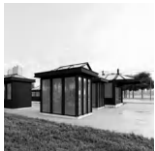
Public Building (Under construction) Modular Metro Entrance. Line 1, 2, 3. (Qingdao, Shandong, China)
