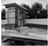
Public Building (Under construction) Metro Elevator. Line 4. (Qingdao, Shandong, China)
