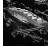
Public Building (Under construction) Metro Station. Line 6. (Qingdao, Shandong, China)
