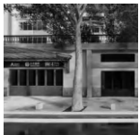
Public Heritage Building (Under construction) Metro Station. Line 4. (Qingdao, Shandong, China)
