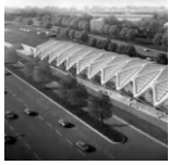
Public Building (Project) Metro Station. Line 6. (Qingdao, Shandong, China)
